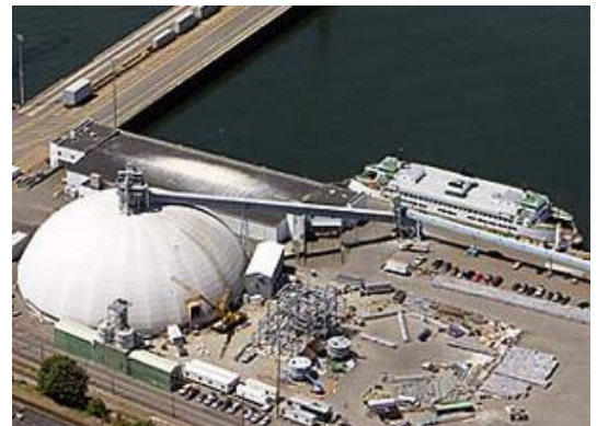
Greenberry Industrial was recognized with a 2007 Northwest Construction Consumer Council (NWCCC) Distinguished Project Award for its work on the Port of Everett, above.
