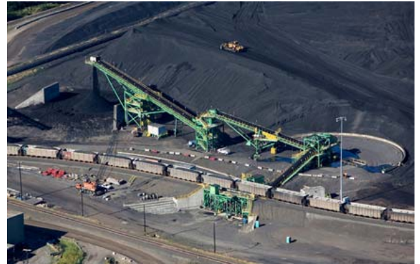
Greenberry Industrial designed and built a new coal unloading system at the TransAlta power plant in Centralia, Wash., that improved efficiency 300 percent.
